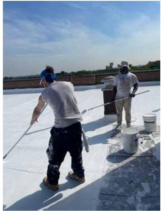
Workforce training participants installing a Cool Roof
